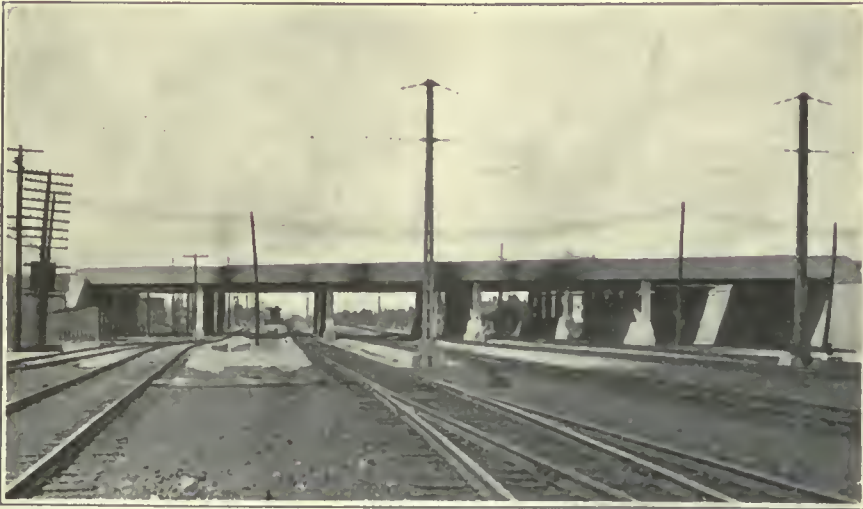
FIG. 267. BRIDGES. Protected plate-girder bridge separating crossing of the Pittsburgh, Fort Wayne & Chicago Railway and the Lake Shore & Michigan Southern Railway from the Illinois Central Railroad, at 75th Street and South Chicago Avenue.
